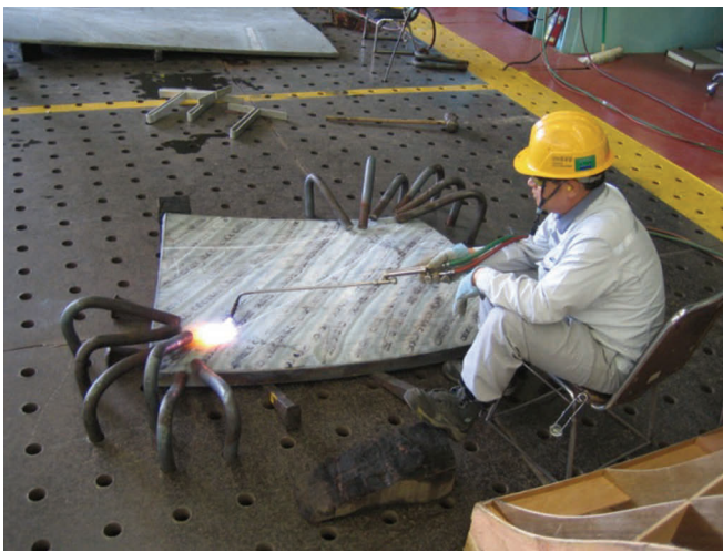
Fig. 4 Thermal bending method by skillful worker (Park, Shin, Ko, Hyun and Doh, 2007).
