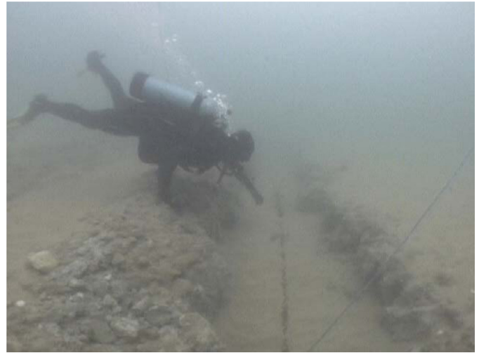
Fig. 2. Cable trench in cemented sediment at dive site 2 in June 2005, approximately 12 months after cable laying. The linear feature in the trench is a measuring tape (Photo: CEE Consulting).
