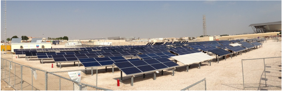
Fig. 1. The 'Solar Test Facility' at Qatar Science and Technology Park, in Doha
