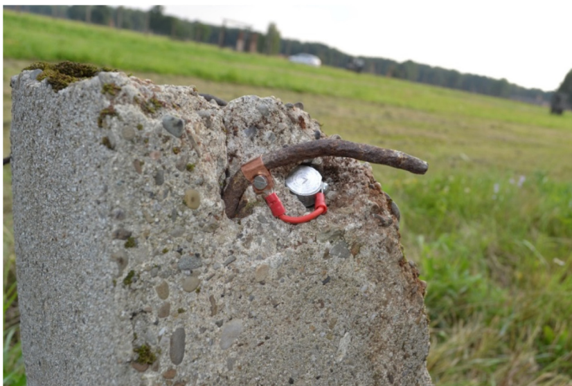
Fig. 7. Pillars located in the former Auschwitz camp protected with sacrificial anodes before applying a new repair mortar: variants with protector buried in soil (a), variant with protector placed directly on reinforcement (b).
