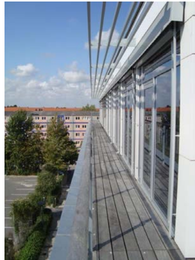
Fig. 4. (a) The stairwells are much brighter after the concrete facades have been replaced with glass facades. All windows are made with sunscreen to limit overheating; (b) The penthouse has both vertical and horizontal solar shading to avoid high indoor temperatures during summer.
