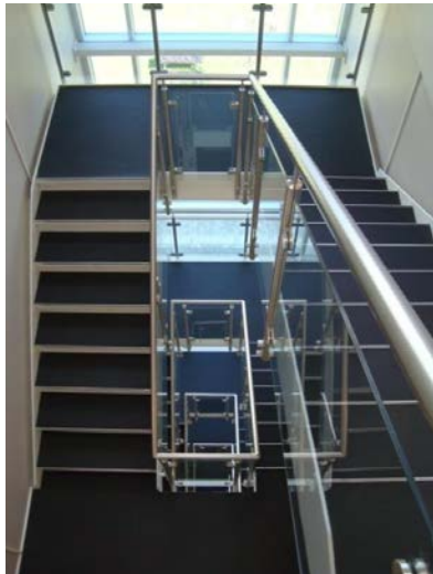
Fig. 4. (a) The stairwells are much brighter after the concrete facades have been replaced with glass facades. All windows are made with sunscreen to limit overheating; (b) The penthouse has both vertical and horizontal solar shading to avoid high indoor temperatures during summer.
