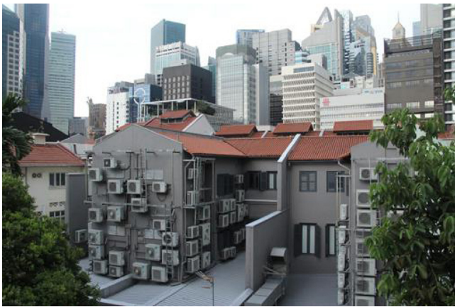
Fig. 1. Typical installation of split unit condensers in a crowded and hidden location.
