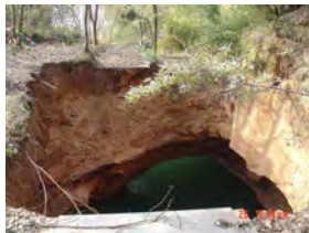
Fig.53 New roof rock collapse with a plane area of 75 m 2 of the originally partially failed rock cavern No.24.
