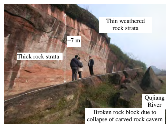
Fig.41 Rock mass profile exposed due to collapse of a carved rock cavern on Qujiang River about 3.5 km west to the small hill site.
