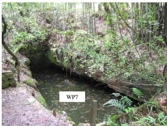
Fig.3 A small water pool of 12 m long and 2 to 5 m wide for vertical portal of the immersed rock cavern No.7 on the small hill.
