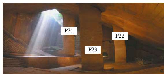
Fig.4 Unwatered rock cavern No.2 with four rock pillars, one rock staircase, one vertical portal with sunlight and curved imprints on the rock surfaces of sidewalls, three pillars (P21, P22 and P23) and inclined roof in argillaceous siltstone of Cretaceous age.
