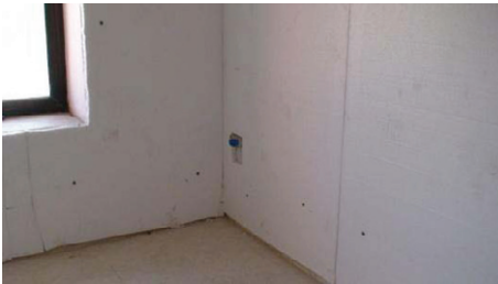
Fig .3 Thermal insulation boards for walls
