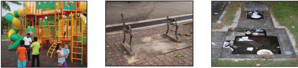
Fig. 3. (a) This new children playing equipments are in good conditions but the playground is located beside a main road; (b) Street furniture in bad condition and dangerous for the kids and toddlers. This is due to acts of vandalism. This is located the playground near the low cost apartments. (c) The drains surrounding the open space area are not closed thus prone to be filled with rubbish, smelly and dangerous. It is also an eye-sore.
