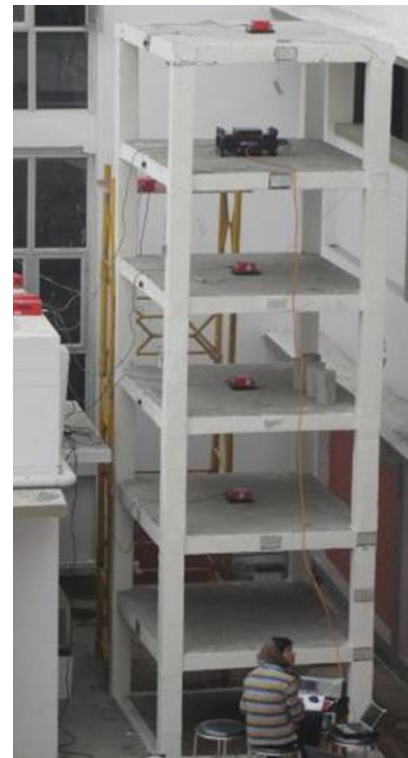
Fig. 1. Scale down six storey RC building constructed and monitored for health monitoring studies
