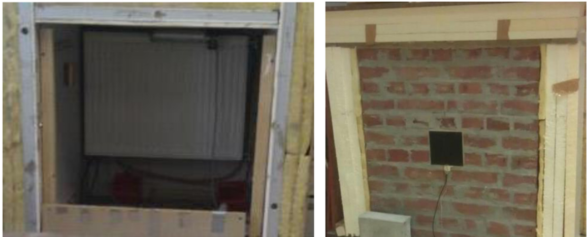
Fig. 2. Experimental setup of the wall and the heating box.
