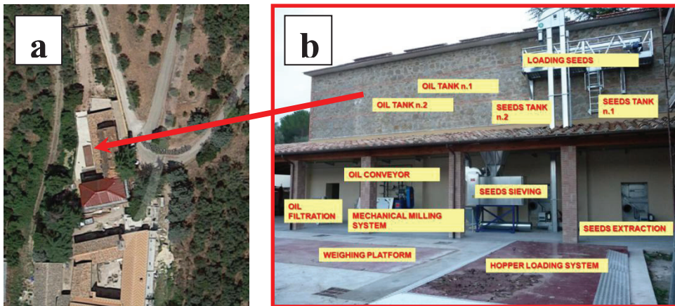
Fig.1 (a) Aerial view of the case study location; (b) vegetable oil pilot plant and its components.
