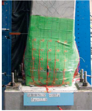
Fig. 10. PET jacket without fracture in hinge zone.
