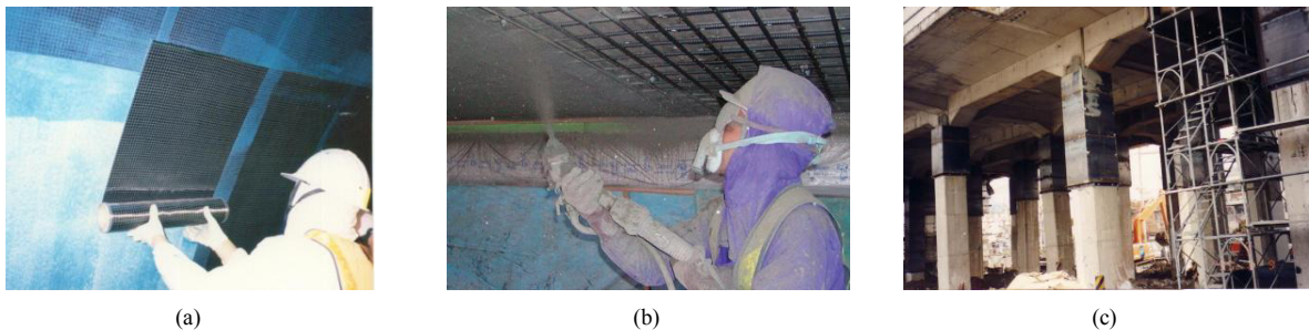
Fig. 1. Three types of strengthening, (a) External bonding, (b) Overlaying (spraying), (c) Jacketing
