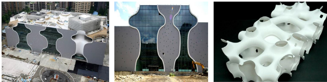
Figure 5 (left-middle) The opera house at finishing stage. (right) A model for the opera house. Source: http://uk.phaidon.com/agenda/architecture/articles/2014/September .
