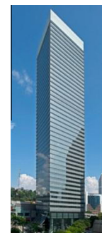
Figure 3. Case study building.
