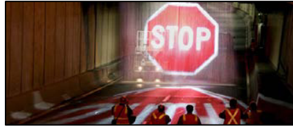
Fig. 4. Laservision, pseudo-holographic warning sign.
