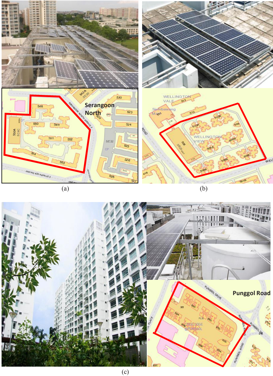
Fig. 1. (a) Solar PV test-bedding at Serangoon; (b) Solar PV test-bedding at Wellington; (c) Treelodge@Punggol. The three precincts were installed with monocrystalline panels.
