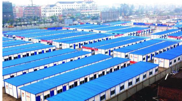
Fig. 1. One post-disaster transitional settlement of prefab houses in Wenchuan earthquake
