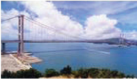
Figure 5. Hong Kong Tsing-Ma bridge
