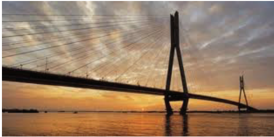
Figure 1: No.2 Nanjing Yangtze River Bridge
