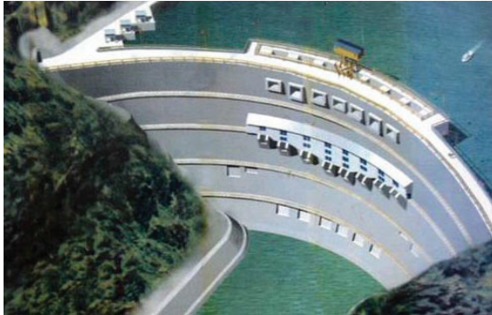
Figure3. Xiluodu arch dam
