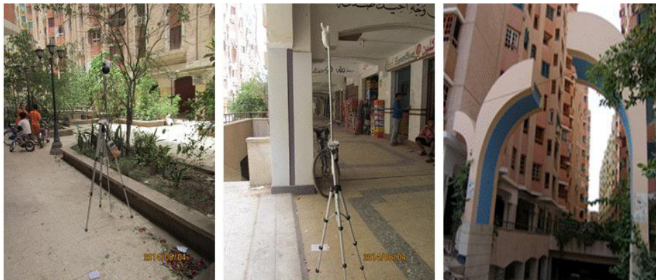
Fig. 4. The overall view of the outer courtyard of El-Abrahimia and El-Moalemen complexes.
