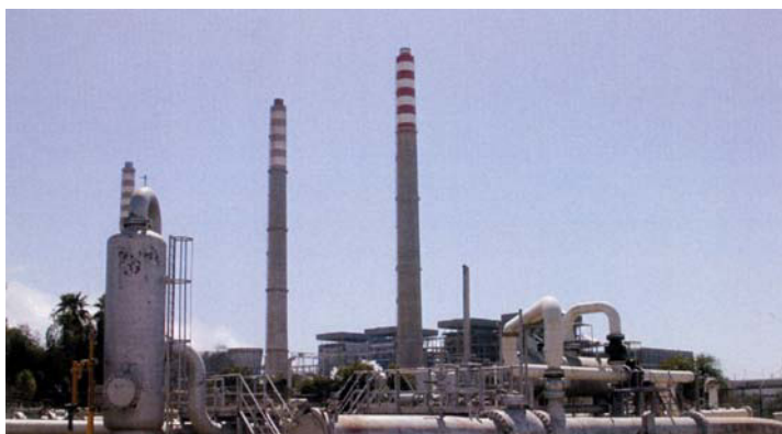
Figure 4. A picture of Ramin power plant near Ahwaz
