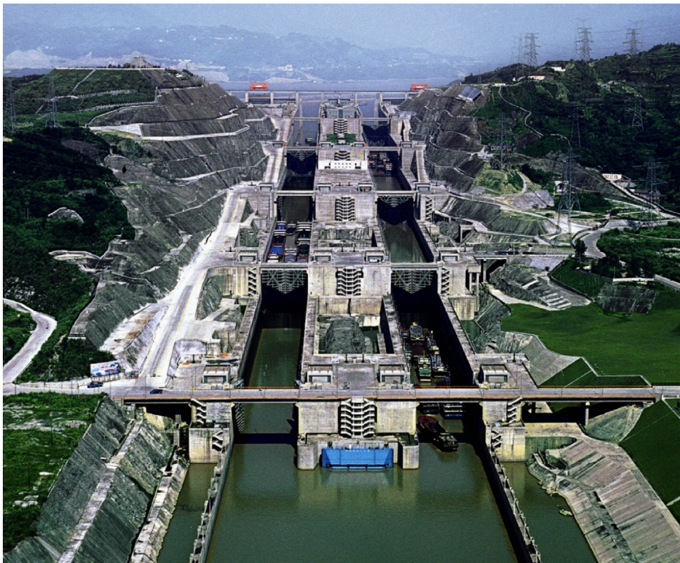
Fig. 2. Photo of the high slope of the double-lane five-step ship lock of the TGP.
