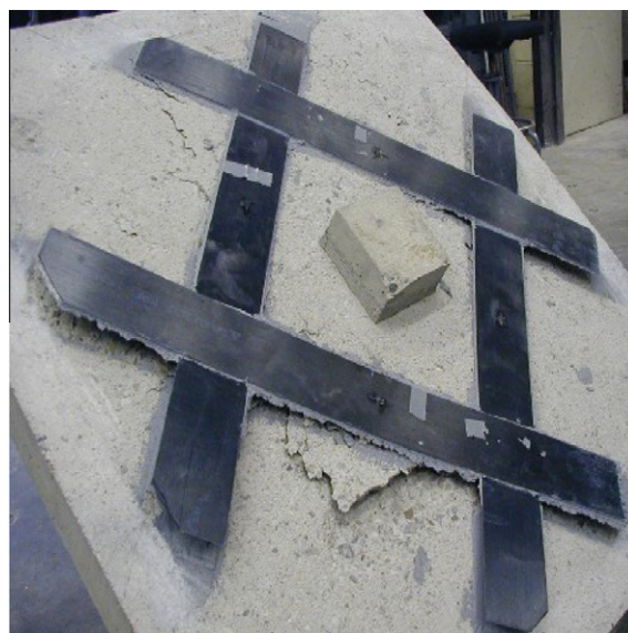
Figure 5 Punching shear failure cracks on slab S-4-S-O (bottom face).
