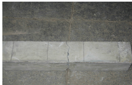
Plate 4 Cracking Pattern of Prism Specimen
