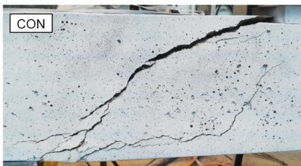
Fig. 7. Dominant shear crack in the control beam.
