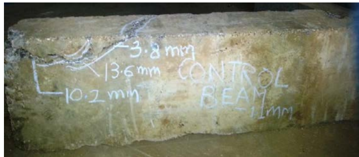
Fig 6 Crack width of control beam
