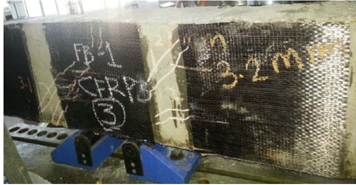
Fig 8 CFRP bonded RC beam1 (CFB1) after testing
