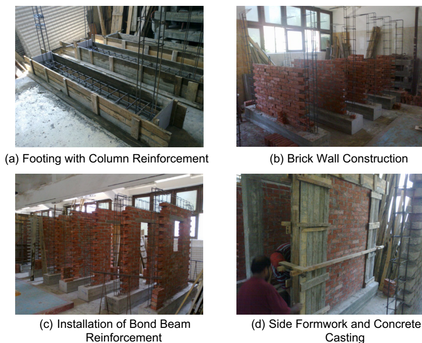
Fig. 2 Construction sequence of the wall assemblies.
