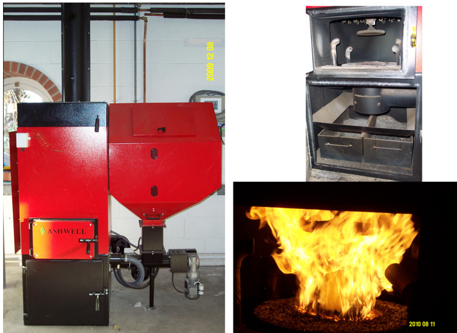
Fig. 4. 50 kW th wood pellet boiler and its combustion chamber and flame.
