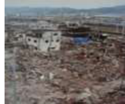
b) Hanshi-Awaji Earthquake
