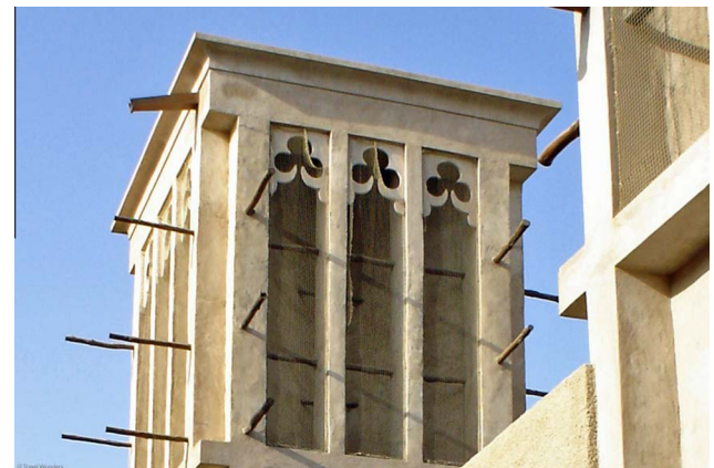
Fig. 4 Traditional wind tower in Gulf states. Steele, James [16].
