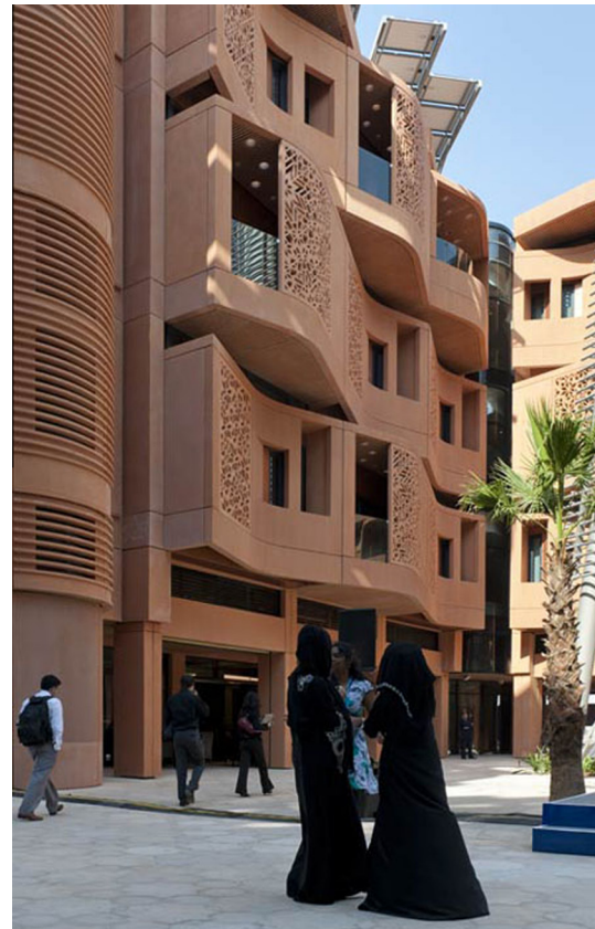
Fig. 15 The main housing courtyard. www.masdar.ae/
