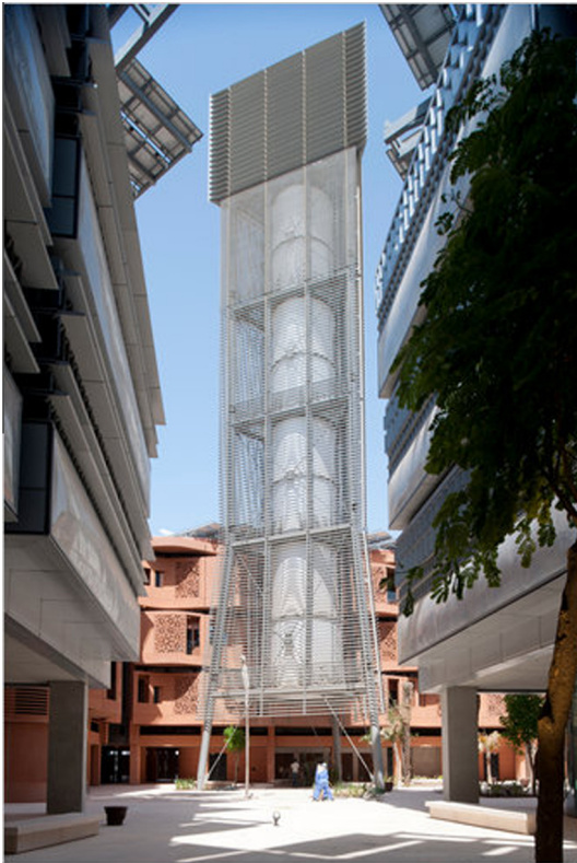
Fig. 14 Wind tower in the housing courtyard. www.masdar.ae/
