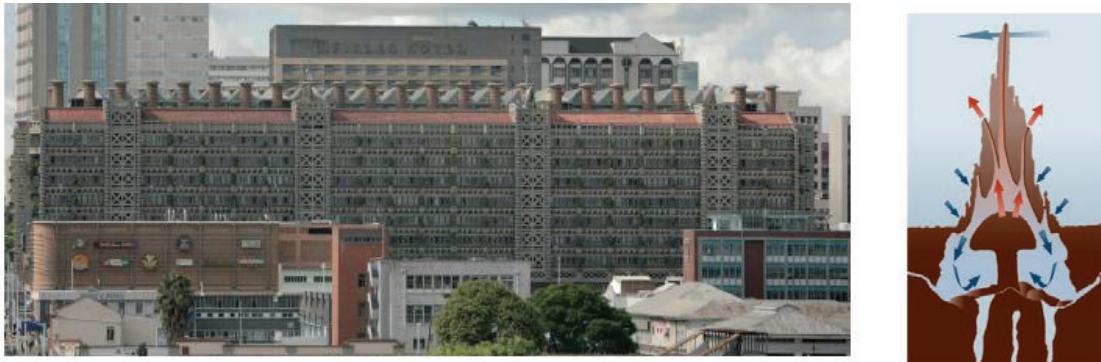
Fig.4. On left (Eastgate Building in Harare, Zimbabwe); on right (schematic of termite mound).
