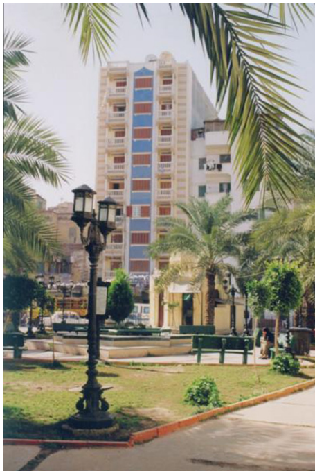
Figure 15 An example of the bold new developments introduced inside “Abu al-Abbas Square” area, which was designated under the Act No. 106 as “Streets and Areas of Restricted Building Regulations”. This example reflects the inefficiency of the designation as “Streets and Areas of Restricted Building Regulations”, regarding that the maximum allowed building height inside this area is 16 m [45].
