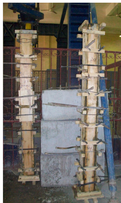
(b) Formworks for column specimens of group2
