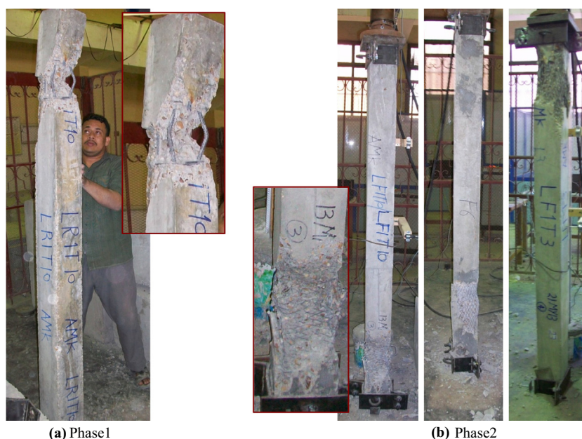
Figure 14 Failure of column specimens of group2.
