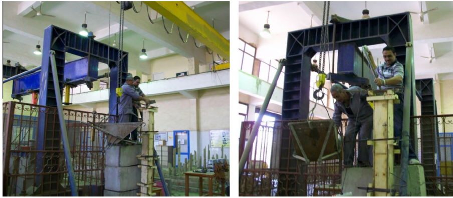
Figure 4 Casting and vibrating of concrete.
