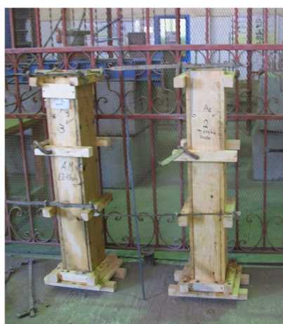
(a) Formworks for column specimens of group1
