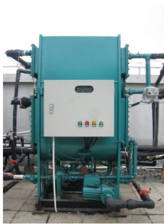
Fig. 2. LiBr/H 2 O single-effect absorption chiller
