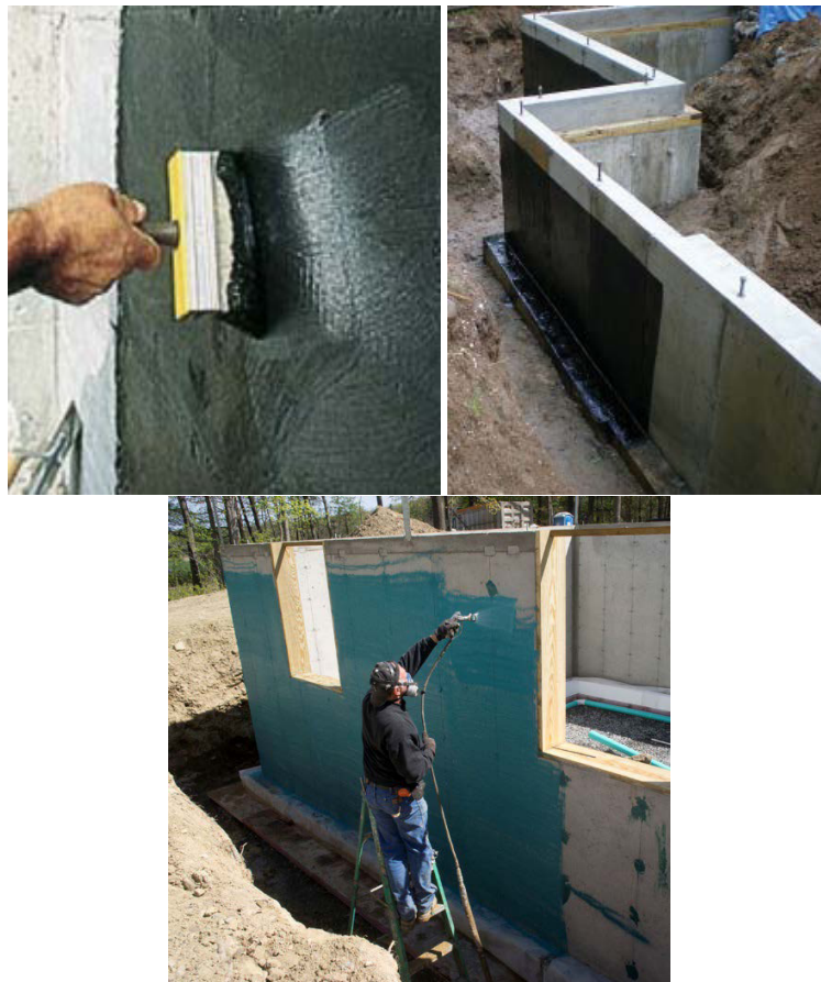
Fig. 2. Application of bitumen emulsion (first and second image) and of polymer emulsion
