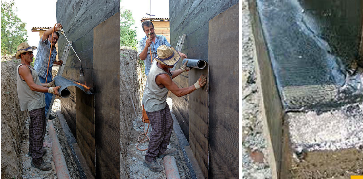
Fig. 3. Application of bitumen strip insulation
