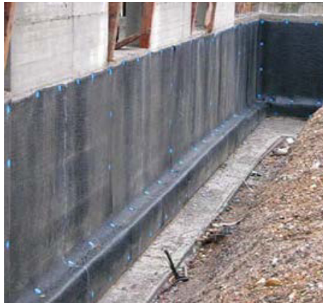
Fig. 6. Insulation of a building using bentonite hydro-insulation
