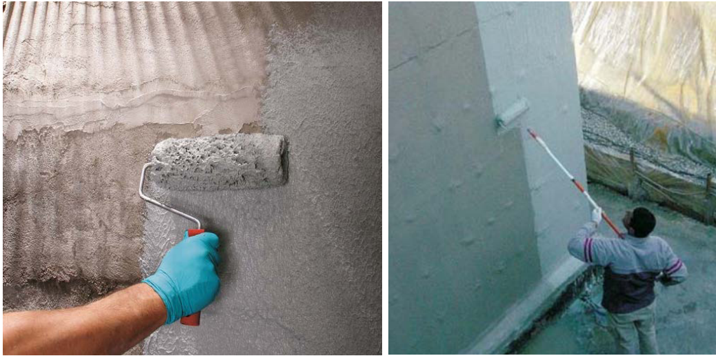
Fig.5. Hydro-insulation cement mass used for insulation of the dug-in building
