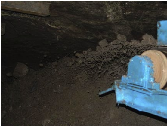
Fig. 6. Backfilling technology underground
