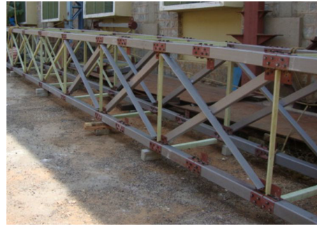
Fig.3. Photograph showing pultruded connection on a composite tower
