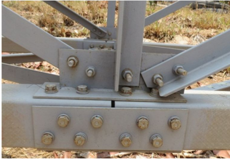
Fig.2. Photograph showing leg member joint
