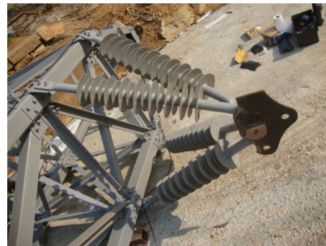
(b) Connections at base portion of the cross arm.
