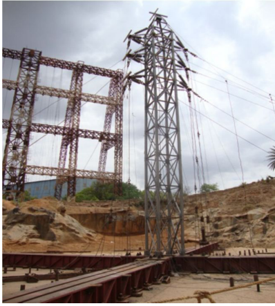
Fig. 4. Rigging arrangement of composite tower on the tower test bed
