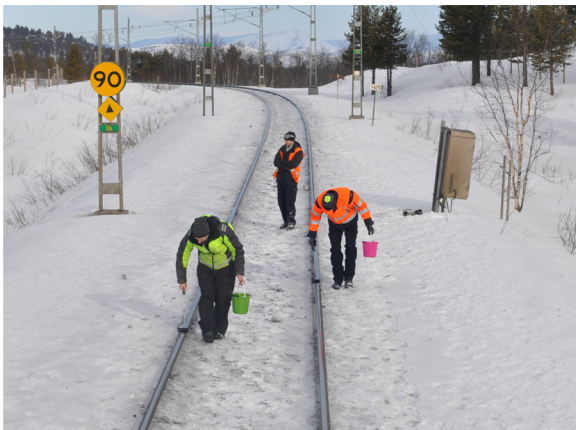
Fig. 4. Method for applying the ToR friction modifier.
