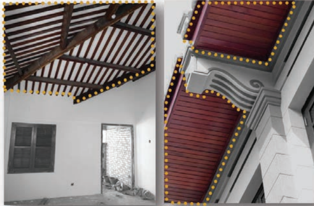
Fig.8(a) and (b) Timber for purlin and fascia
