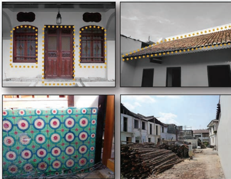
Fig.9(a), (b), (c) and (d) Reused material such as window and door, roof tile, Indian tile, and also timber
