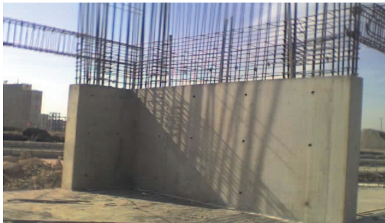
Figure 1: Flanged section shear wall.
