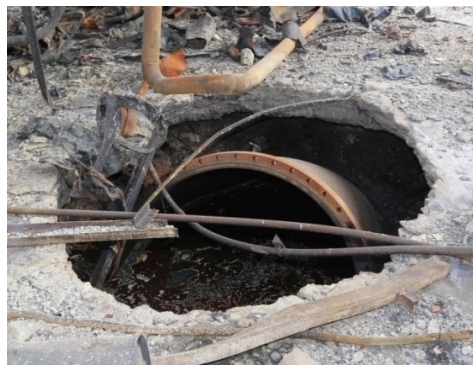
Fig. 2. Lower part of the reactor.
