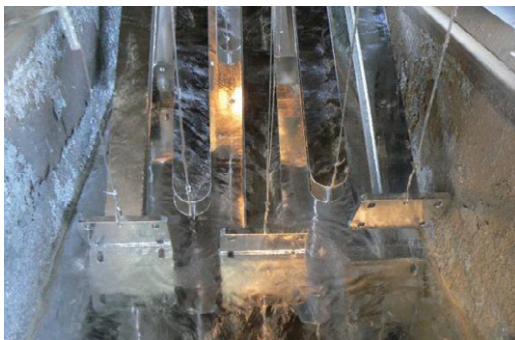
Fig. 1. Hot dip galvanizing of prefabricated load-bearing steel components
