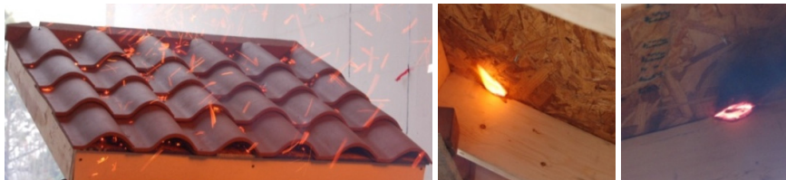
Fig. 2. Images of experiments conducted using oriented strand board/ceramic tile (OSB/CT) without bird stops installed [32]. Intense smoldering ignition (SI) was observed within the OSB base layer and eventually flaming ignition (FI) was observed. The wind tunnel speed was 7 m/s and the Firebrand Generator was located 2.0 m from the CT roofing assembly. The dimensions of the roof assembly were 122 cm by 122 cm.
