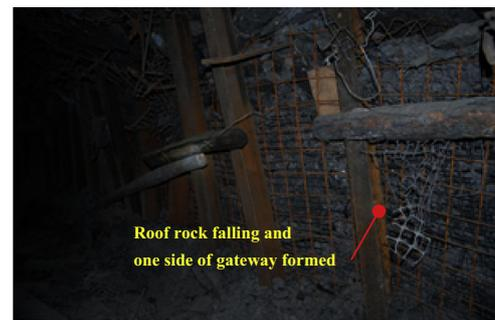
(a) Steel and mesh support for cracked roof falling.
