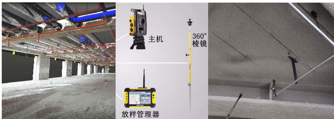
Fig. 2. Point cloud model combined with robotic total station layout
