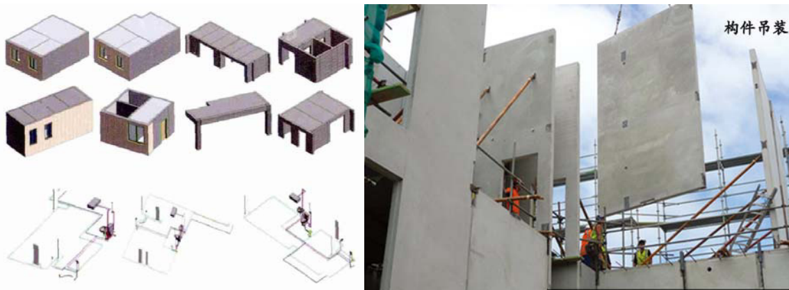
Fig. 1. Modules at different level and the on-site erection of components
