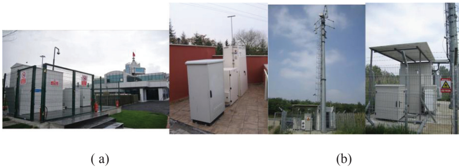
Fig. 5. Fuel cell back-up power systems in (a) daily operations and (b) telecommunications towers
