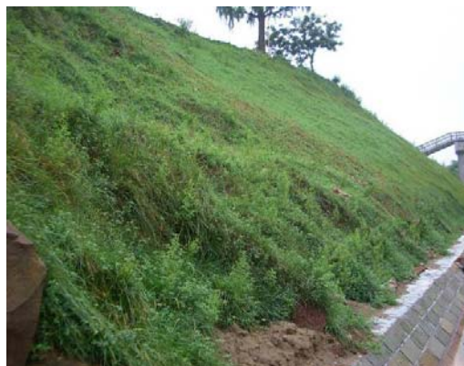
Fig.7 6 months after completion
