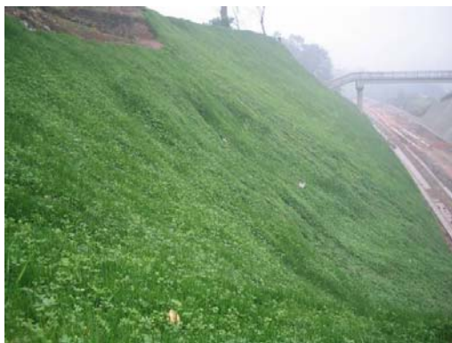
Fig.7 3 months after completion
