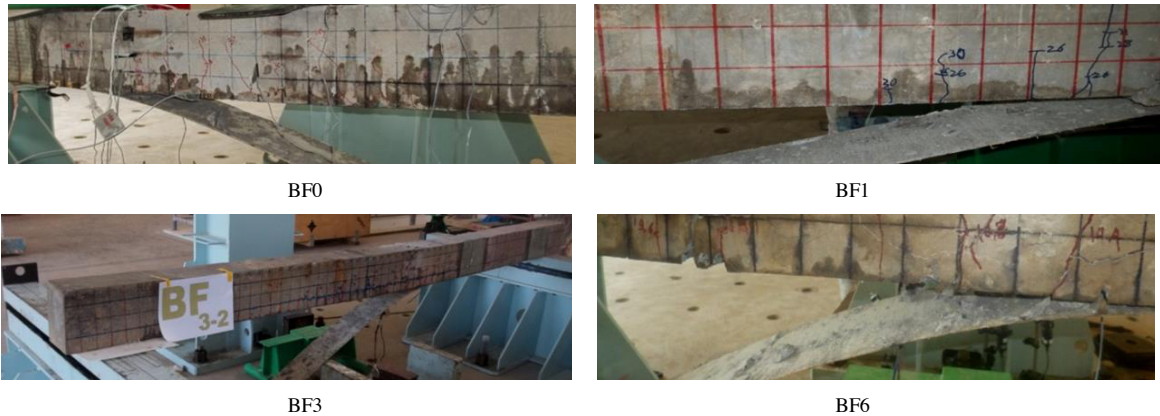
Fig. 8. Failure mode of the beams
