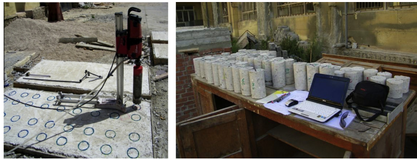
Figure 7 Core drilling at pre-specified locations and some extracted cores.
