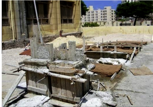
Figure 8 General view for columns and slabs.
