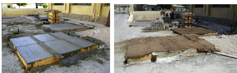
Figure 6 Some reinforced concrete slabs used throughout the program.
