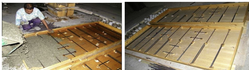
Figure 3 Reinforced slabs with different configurations of reinforcement and depth.
