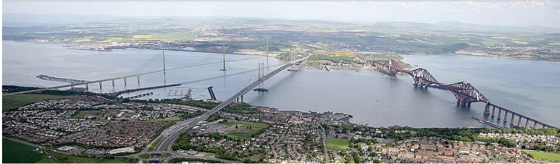
Figure 1: Visualisation: Three centuries of engineering in the Firth of Forth
